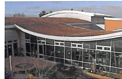
Roof designs on new schools often have concealed gutters and projecting aerofoil fascias. These soften the lines of the building and accentuate curved frontages.
